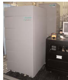
Nuvera’s Avanti fuel cell power module is helping JGA to develop PEM fuel cell codes and standards for the Japanese market.
